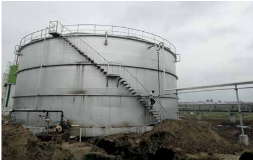
Picture 4: A visual of continuously stirred tank reactor digester of 2,000 m 3
