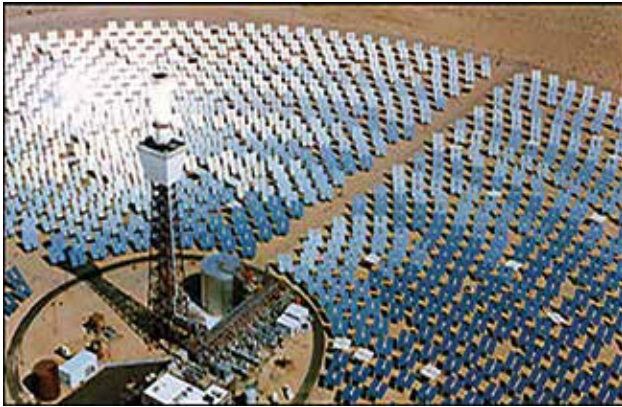
Picture 2: Heliostat with arrangement like sunflower floret
